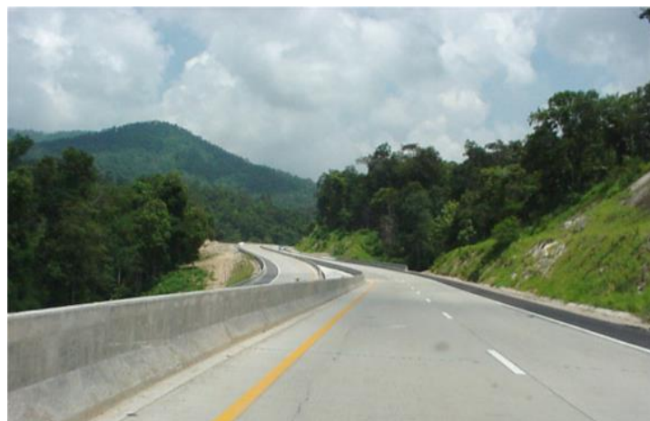
Figure 3.5 Concrete Barrier Median
